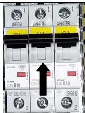
Fig.2 (Q2) Carriage Inverter If you close this switch, power to the carriage's Feed/Brake (carriage's right roller) inverter is closed.
